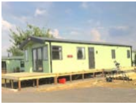
John plumbs it in while Sam builds the deck ...
